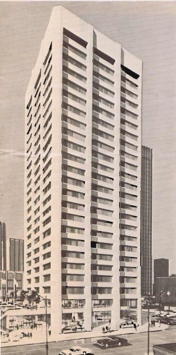
The Standard Life Building, a 26-storey office building being built in Calgary at a cost of $10 million. Architects are Webb, Zerafa, Menkes, with associate architect Anthony Henzell of Calgary. (Photo by Matthews Studio & Photo Lab.)
